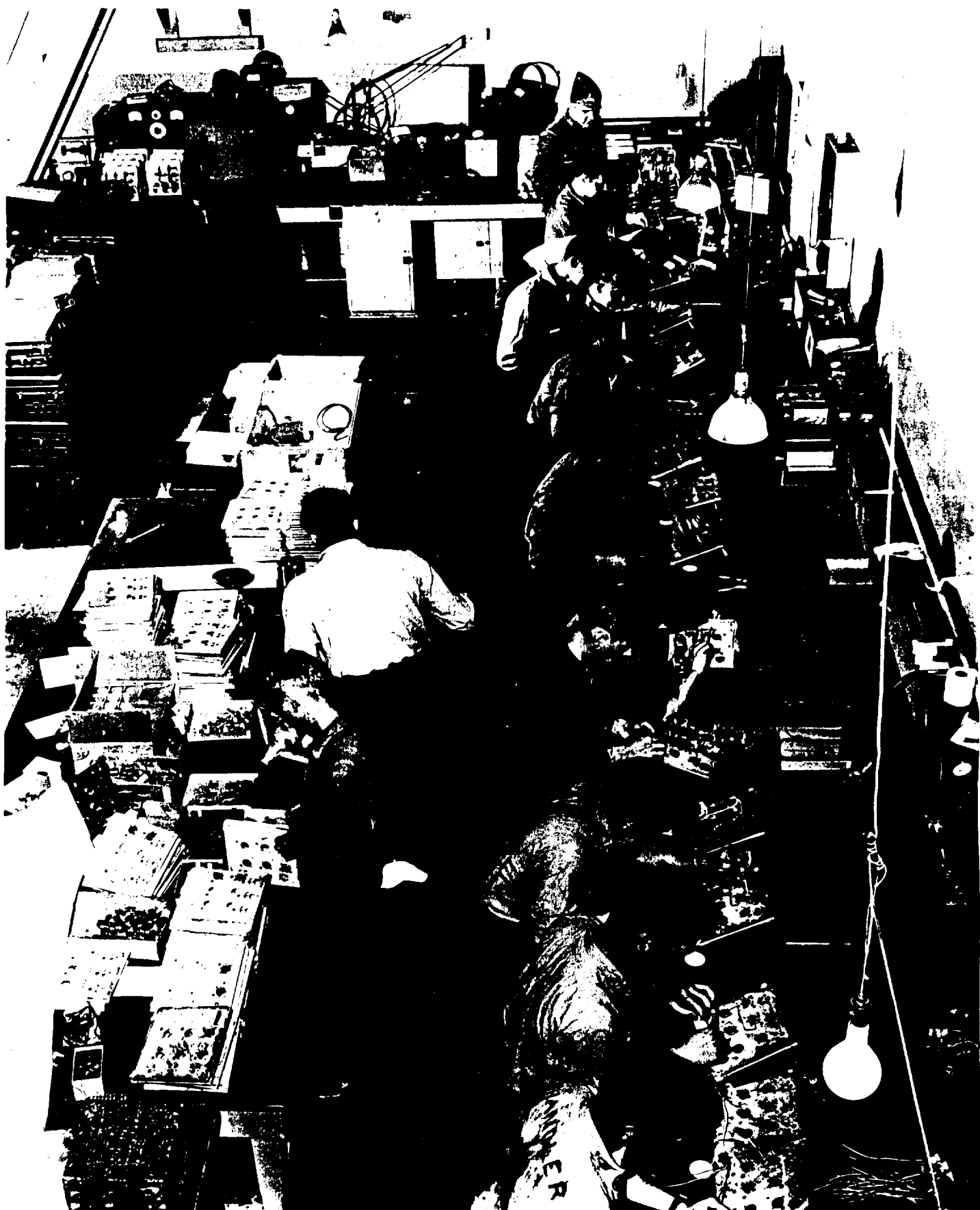
Fig. 24 - Main Timing Unit Assembly Line - Terminal Island
